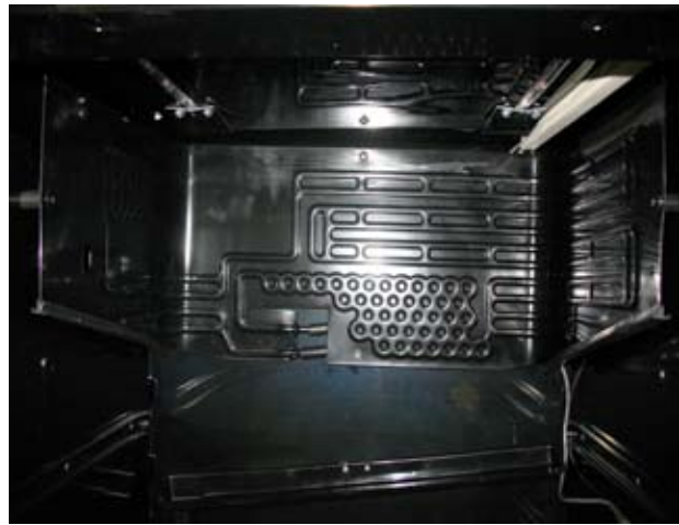
Figure 3.10: U-shaped evaporator plate used in the 61WCM and 6BARM Typical low charge or system leak on this evaporator style will have a frost pattern that is only on the left hand side of the plate, not full across the plate.
